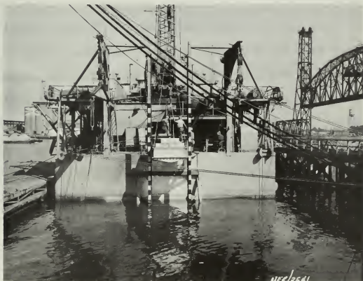
Figure XI-a Model Mounted in Drop Rig Prior to a Test
